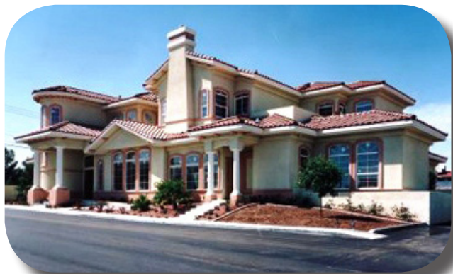
The Ronald McDonald House® in its final construction phase - summer 1998
